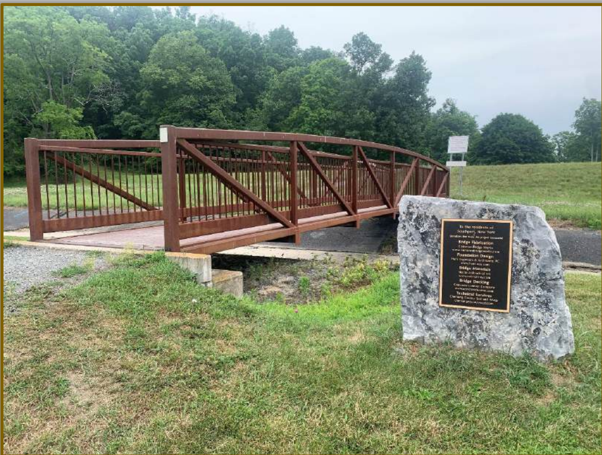
PHOTO 11: PEDESTRIAN BRIDGE AT CHAPEL PARK
