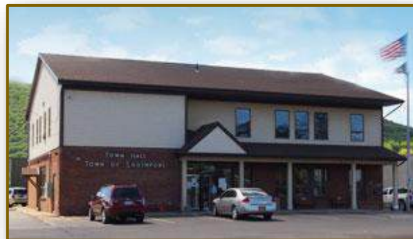
PHOTO 2: SOUTHPORT TOWN HALL
