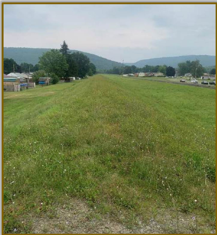
PHOTO 15: LEVEE ADJACENT TO CHAPEL PARK
